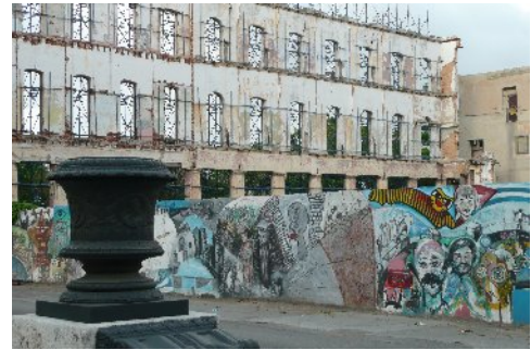
Facade to be saved
