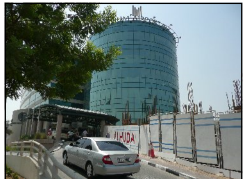
Millenium Hotel and building work
