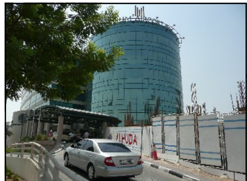
Millenium Hotel and building work
